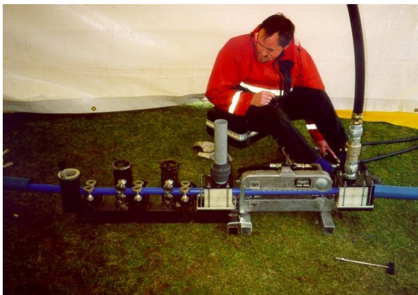
Figure 21. Blowing record 2x1.9 tons of 35 mm copper telecom cable
