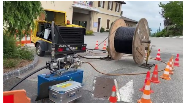
Figure 11. Another commercial cable blowing machine in operation
