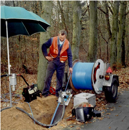
Figure 8. First prototype of cable blowing machine in operation
