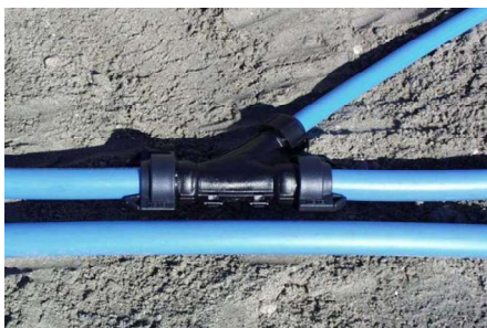
Figure 14. Y-connector branch in microduct networks
