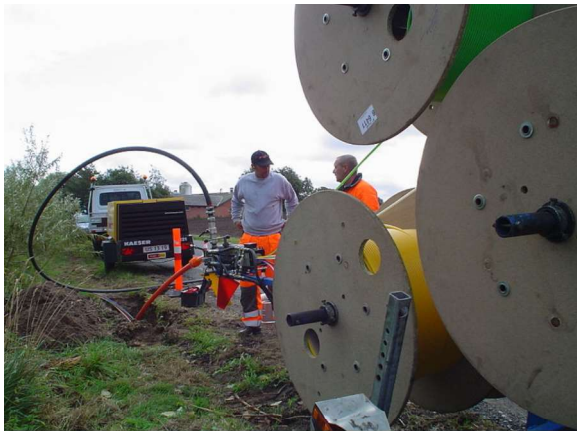
Figure 12. Blowing loose bundle of microducts into a larger duct
